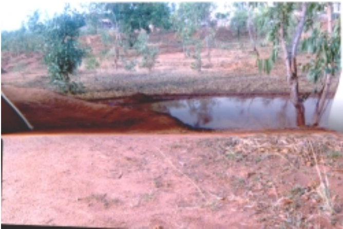
A Contour Trench built by staff and trainees of NISA.
